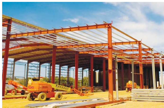
Construction of new DWN Distribution Centre.
