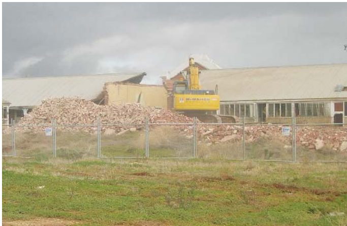
Demolition of Bullring and associated buildings.
